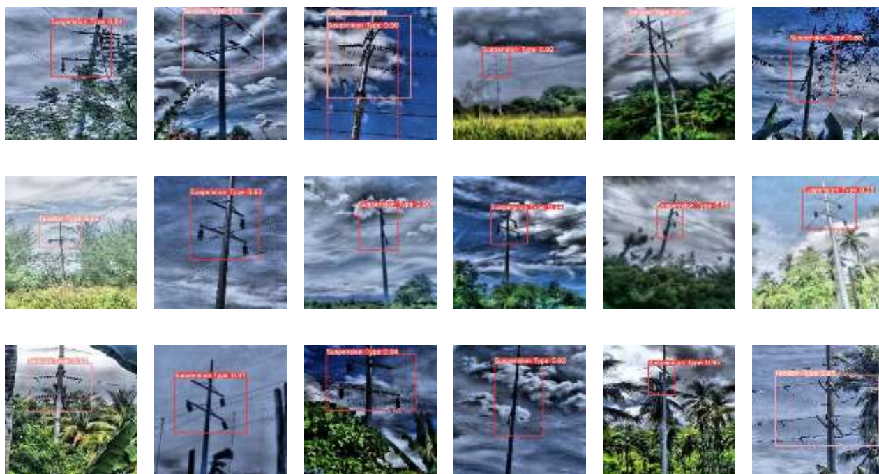
Figure 4. Isolators detected in test images
