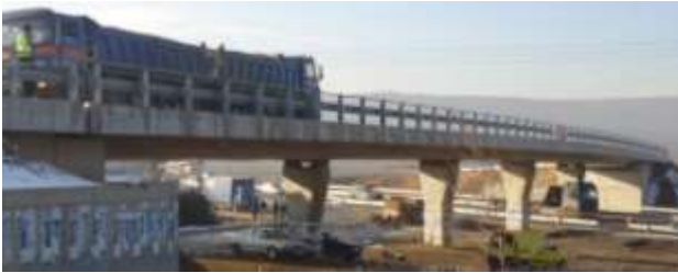
Figure 5. Loaded trucks-Static load position
