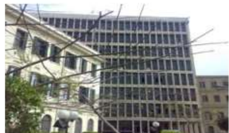
Figure 3. Architecture Engineering Building
