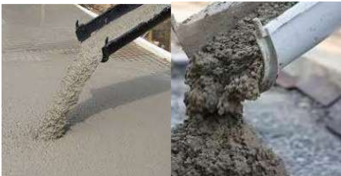
Figure 17: Correct concrete discharge
