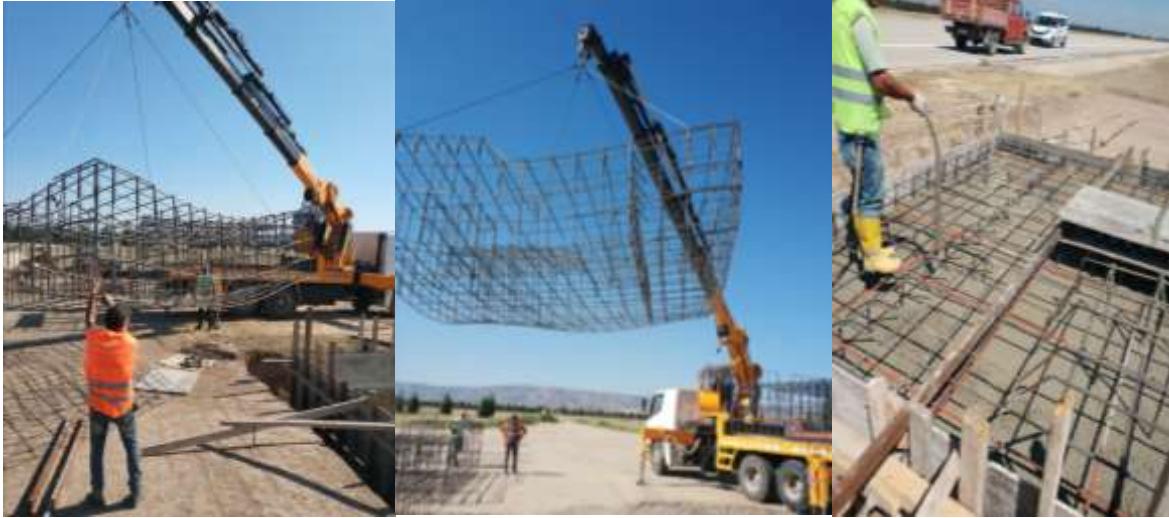
Figure 15: Cage iron-reinforcement transportation process
