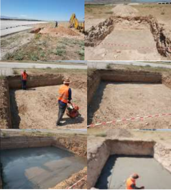
Figure 12: Concreting process of base foundations
