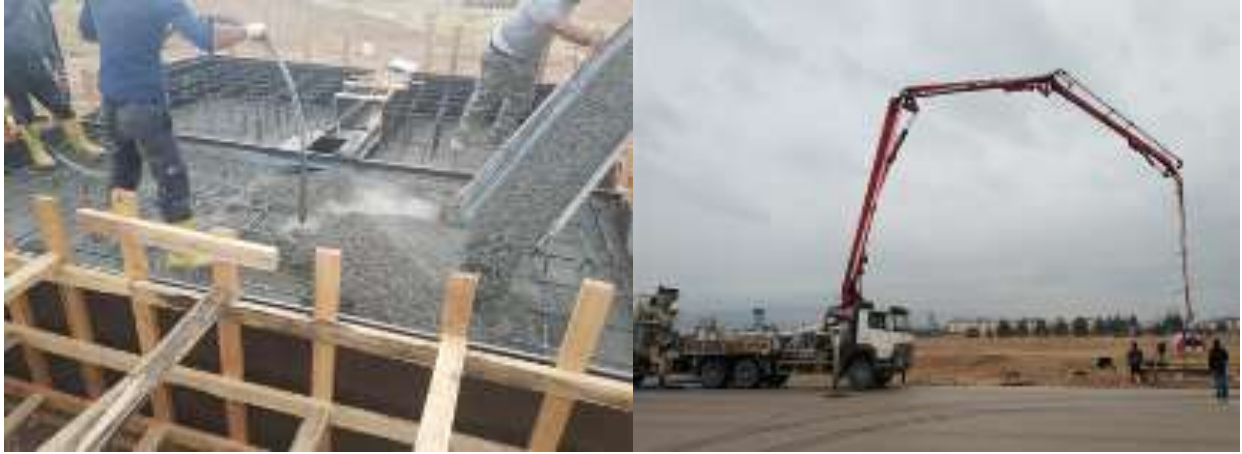
Figure 19: Concrete casting process
