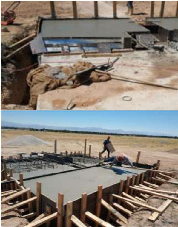
Figure 13: Pedestal foundation concrete formwork controls
