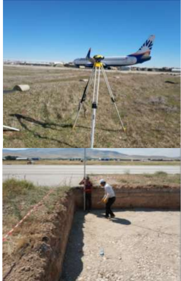
Figure 10: Construction practices of pedestal foundations
