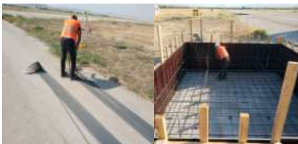
Figure 14: Iron-reinforcement manufacturing at the runway zero point
