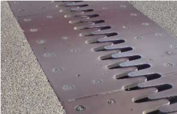
Figure 3. Example of joining two metal plates on a bridge.
