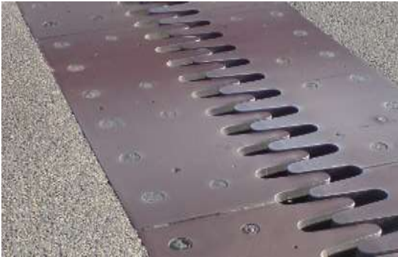
Figure 3. Example of joining two metals plates on a bridge.
