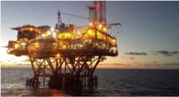
Figure 3. Fixed Offshore Platform View
